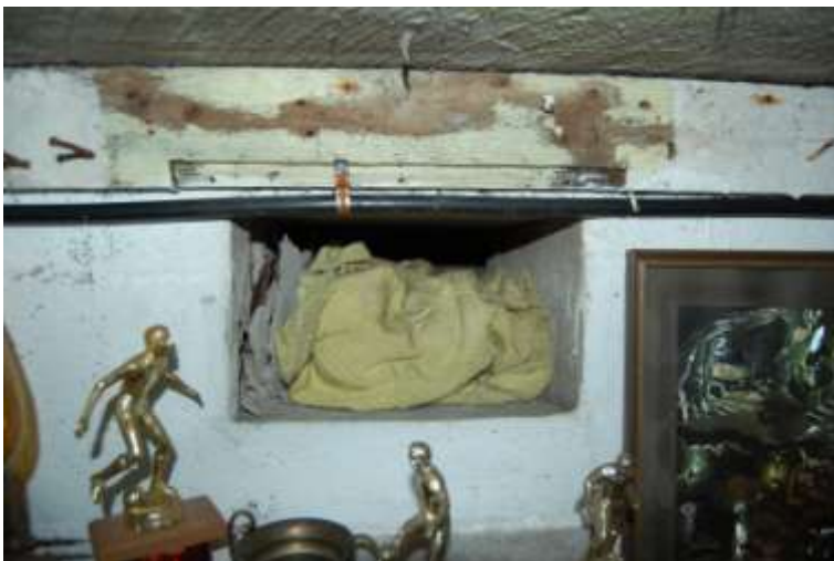
Illus 9 Vent in east wall of shelter
