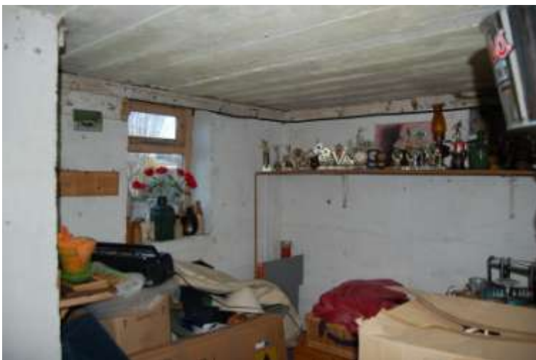
Illus 7 Main shelter facing NE showing Window 1 and shuttering marks on roof
